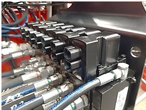
PVED CC, CANopen electric activations mounted on Danfoss PVG32 valve block.
